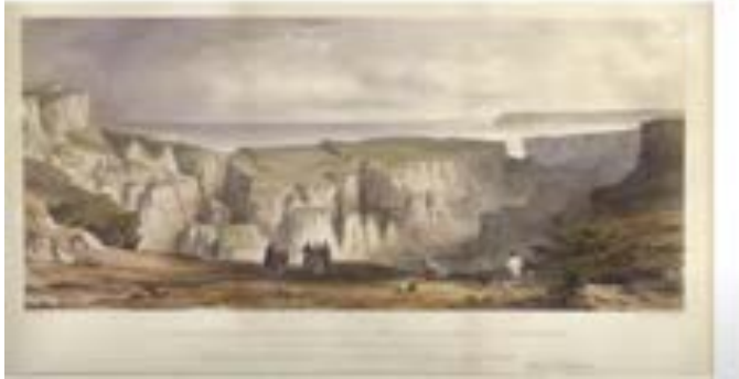
The Great Bindon Landslide
